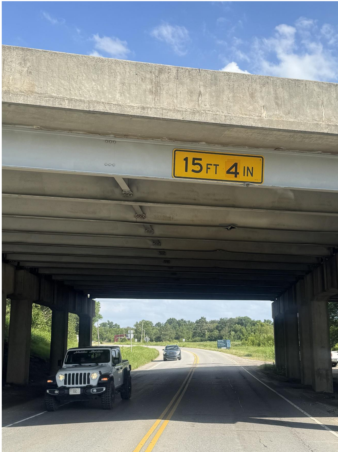
Photo 1: North Edge of Bridge 48.04 Facing North
