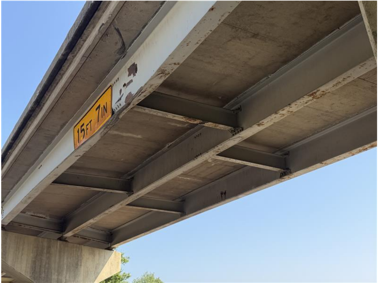
Photo 1: West Edge of Bridge 10.2 Facing East
