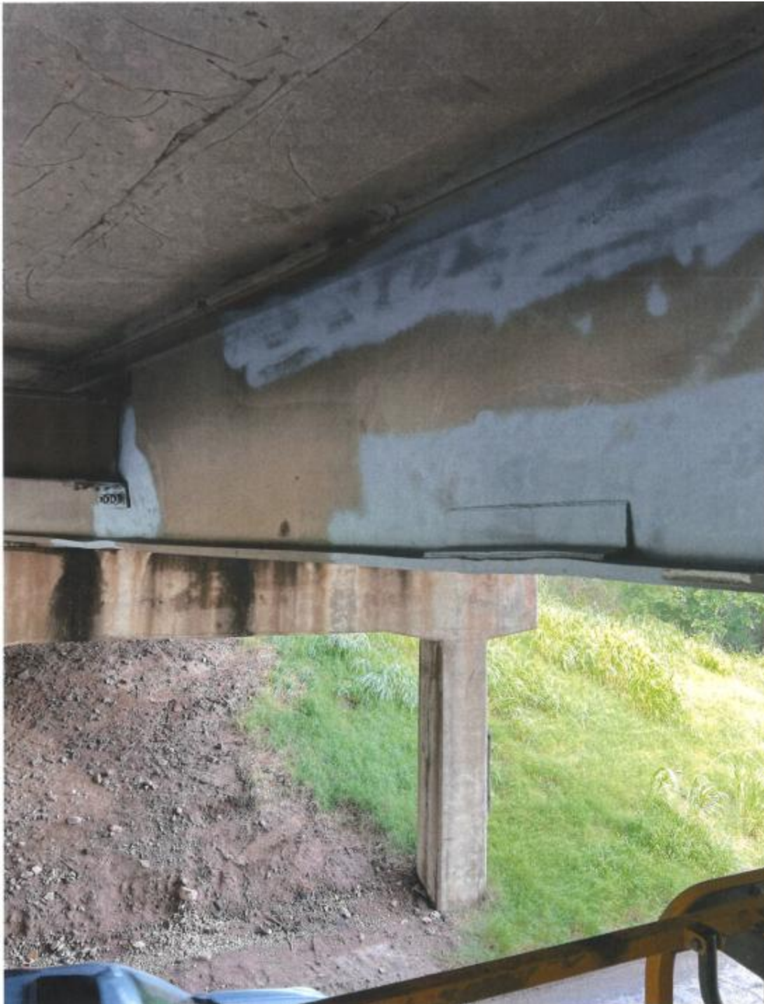
Photo 11: Typical condition of repaired beam
