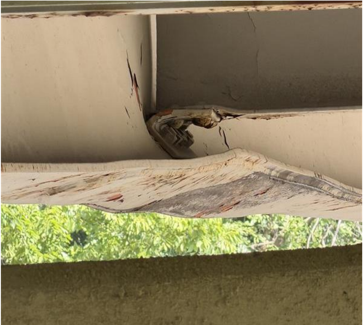
Photo 4: Bent diaphragm web, flange and connecting angle
