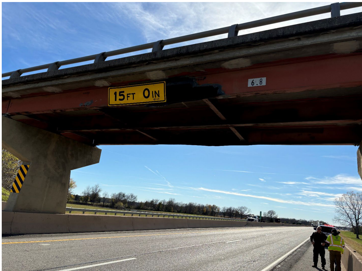
Photo 1 – Bridge Height Clearance Sign
