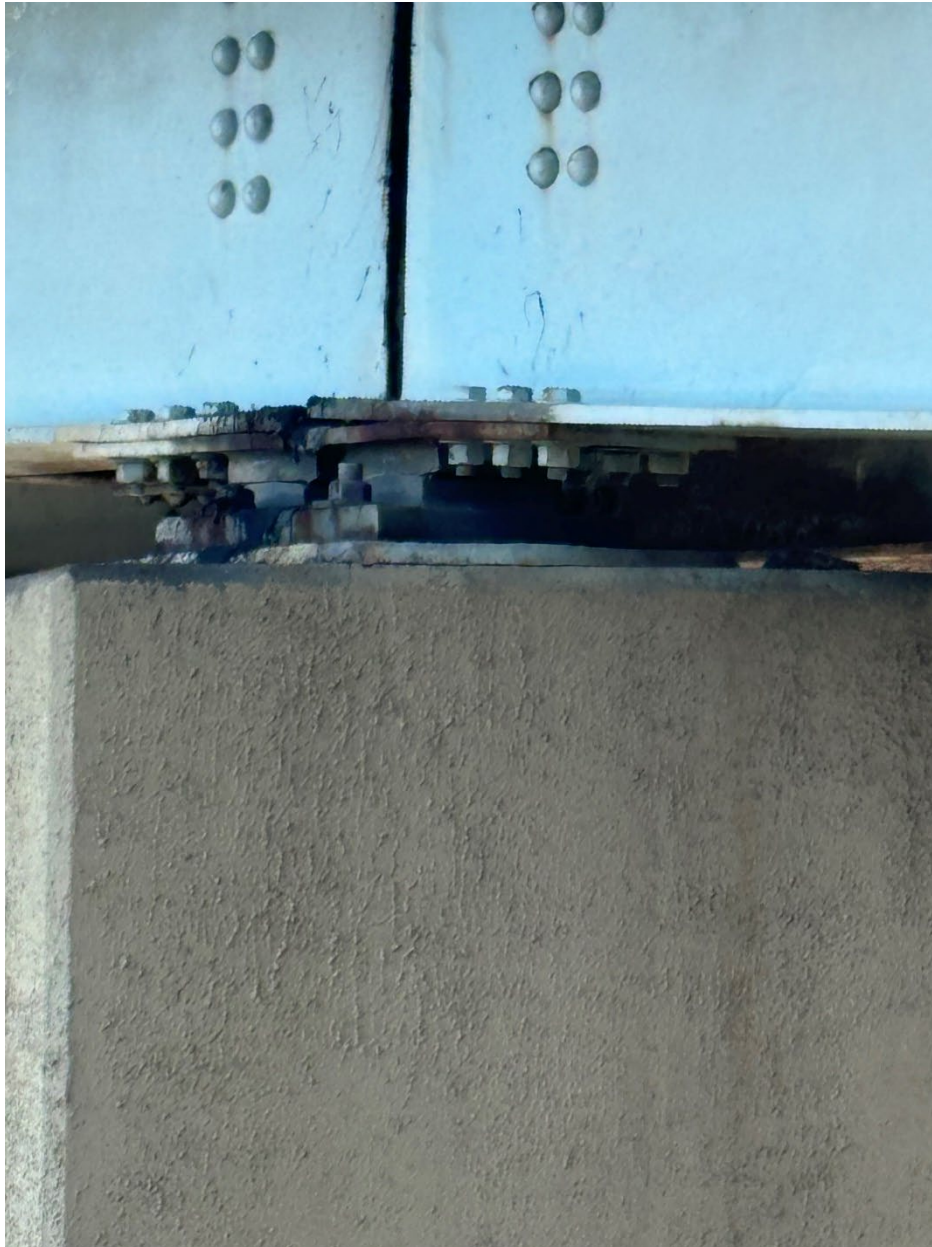
Photo 8 – Typical Bridge Bearing Plates
