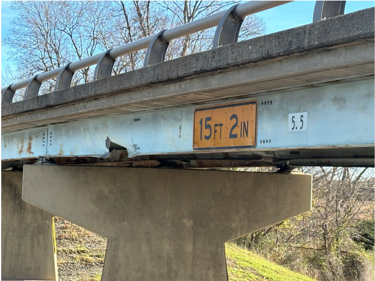
Photo 1 – Bridge Height Clearance Sign
